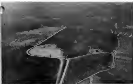
Figure 55. Careless and widespread earth scarring is caused by failure to establish a traffic plan, indiscriminate use of earthmoving equipment, and too much concern with leveling and clearing to facilitate construction. An enforced traffic plan, set up during the planning stage would eliminate much of the revealing scars in this picture.
